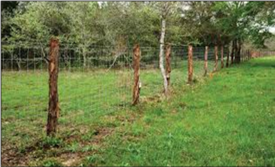
Figure 2.9. An example of a non-electric wild pig exclusion fence built by 50yearfence.com.
